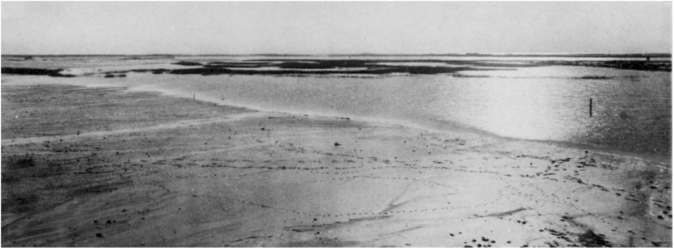
Some idea of the Herculean task of constructing the Lido course is gained from this photograph which shows in the foreground the commencement of the filling process by pumping sand and the water of the lagoons which is now all hard ground
